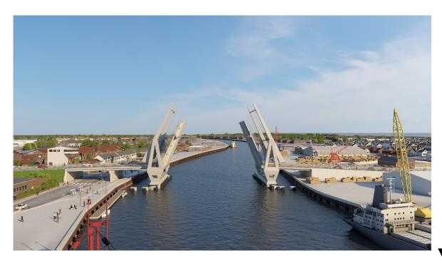
Illustrative example of bascule bridge with counter weights above bridge deck and piers in the river
